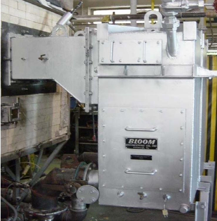
Recent performance testing in China has indicated that using regenerative burners are a viable alternative to conventional hot air combustion, however there are design improvements to the furnace that could be made to improve performance.
