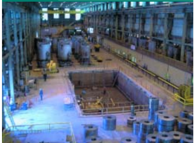
Pit for Phase 1.
