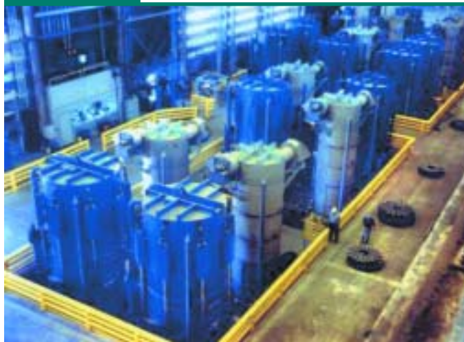
View of the batch annealing facility upon completion of Phase 2.
